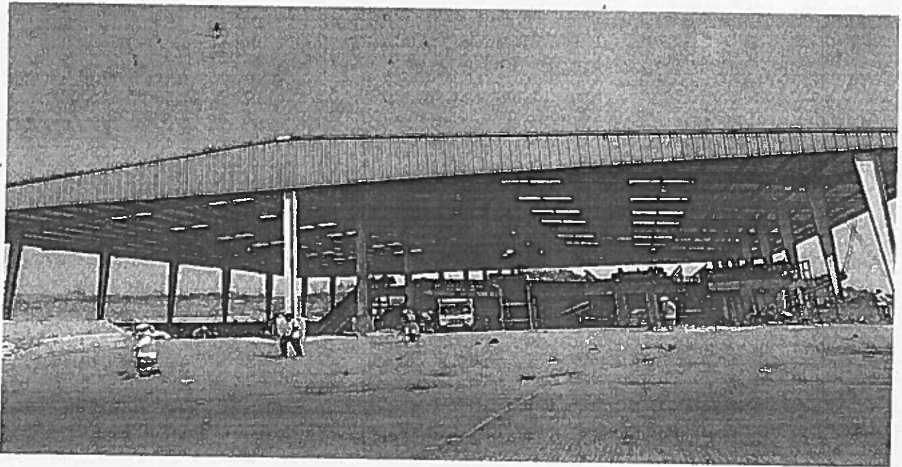
Windrow and Tipping Floor
