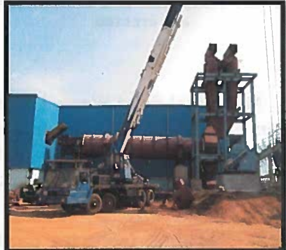
Dryer Erection
