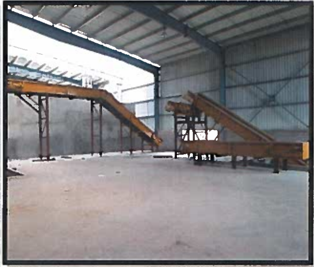
RDF shed - Inner side
