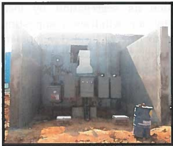
11KV/433V Transformer is erected
