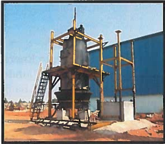
Hot air generator erection
