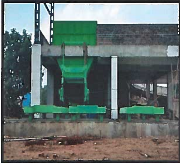
Static compactor and accessories are erected
