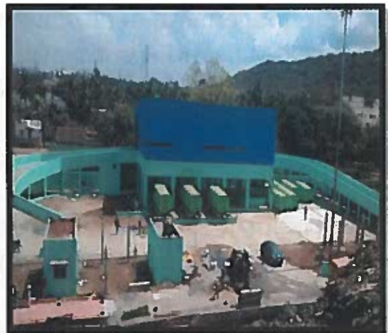
Kannadapalayam Transfer Station
