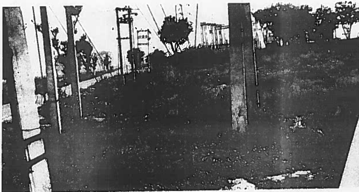
66 KVA Sub-Station adjoining to the site
